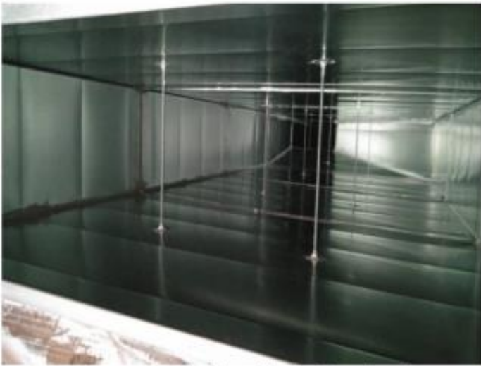
Image 38: Inside of duct after cleaning.
