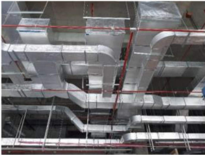
Image 52 & 53: Example of good duct alignment.
