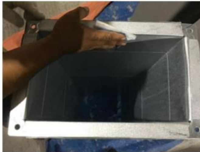
Image 36 & 37: Duct cleaning using IPA.
