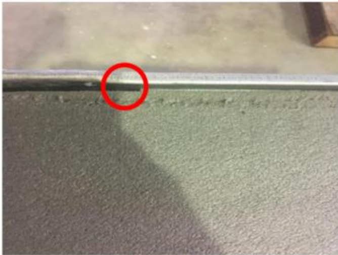
Image 21 & 22: Gap between edge of insulation and duct frame will lead to condensation.
