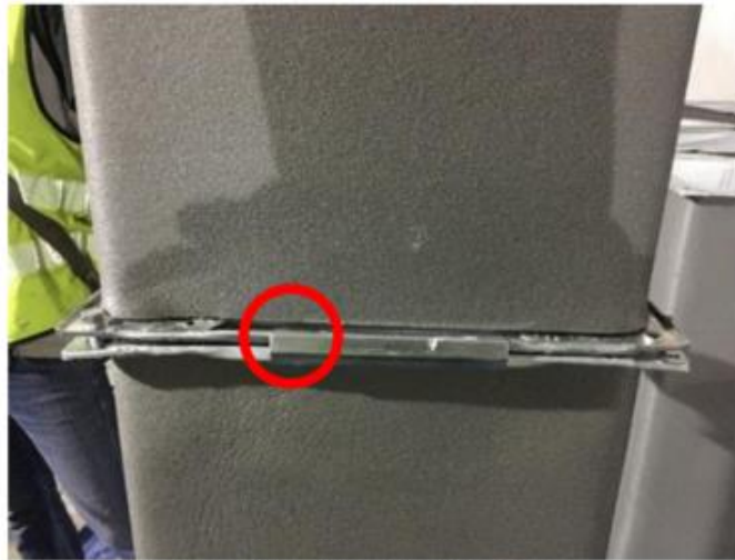
Image 21 & 22: Gap between edge of insulation and duct frame will lead to condensation.
