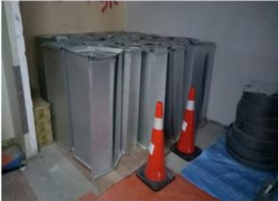
Image 1: Floor covered with plywood.
