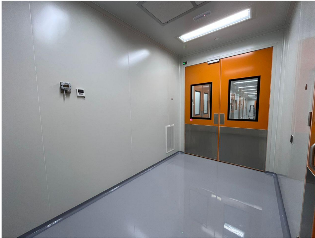
Image 9: Material Airlock In / Out (View 1)
