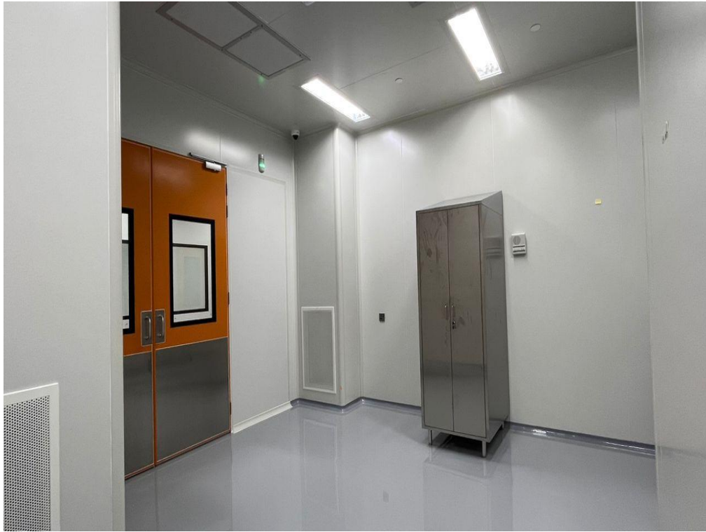
Image 23: Washing / Sterilizing Room (View 2)
