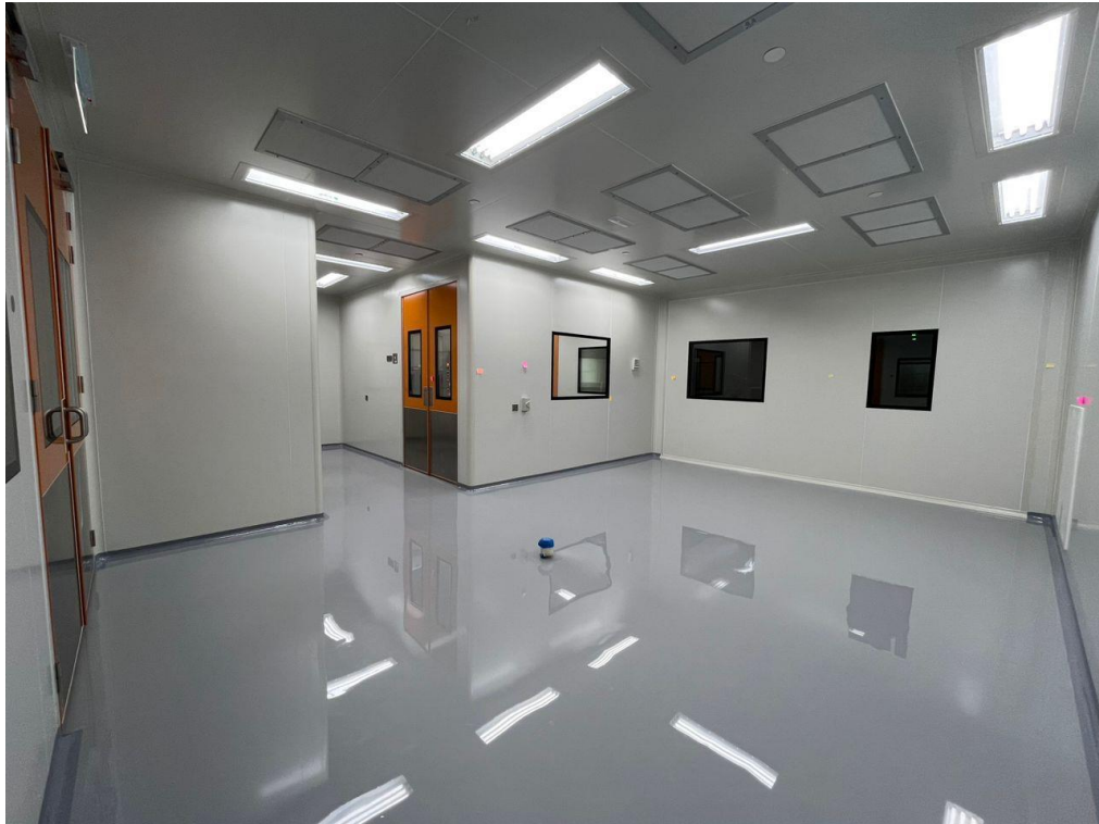
Image 13: Component Preparation Room (View 1)
