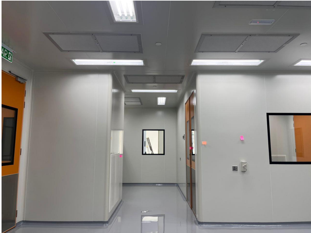
Image 15: Component Preparation Room (View 3)
