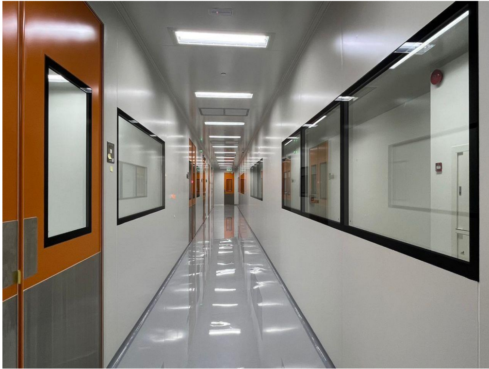
Image 11: Corridor (Grade C) (View 1)
