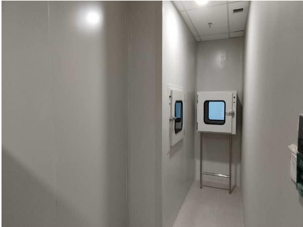
Image 11: Dirty Utility 2 (View 1)
