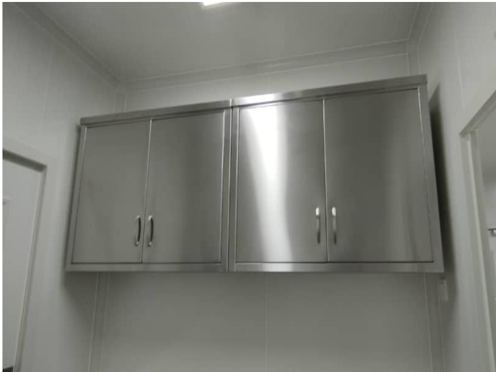
Image 8: Packing & Autoclave Room 2 (View 1)
