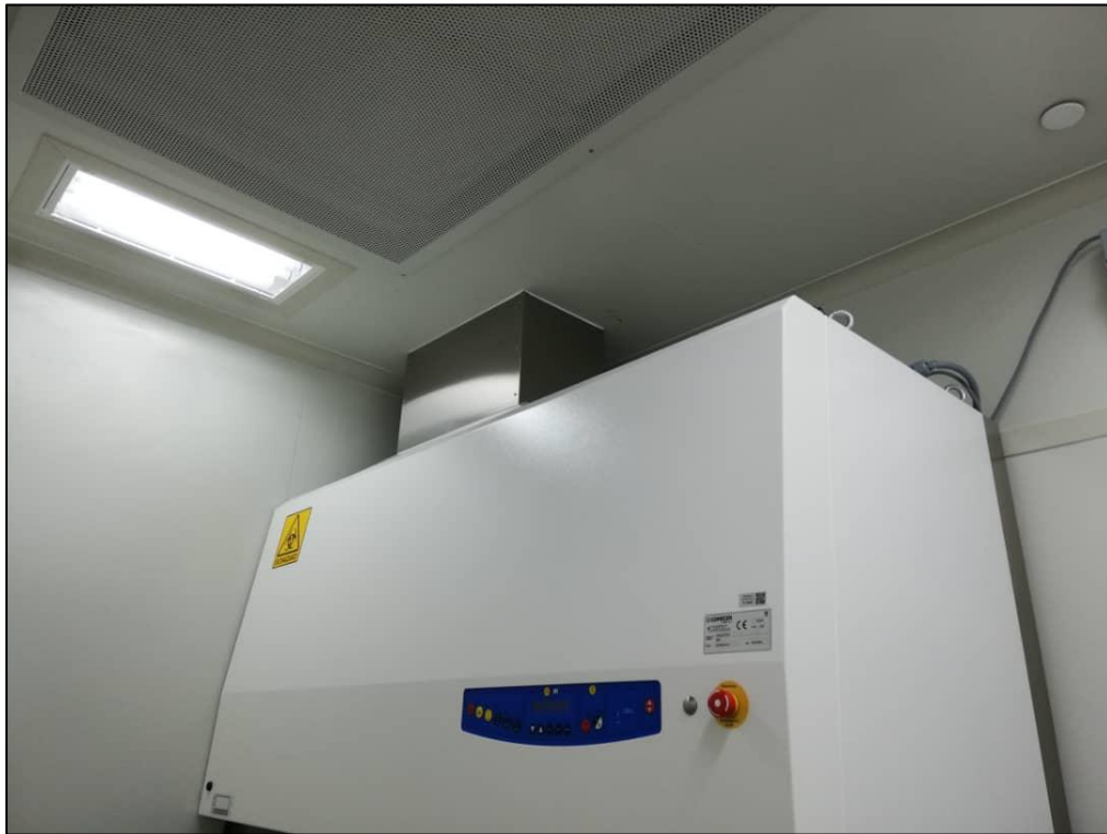
Image 3: SPECT/CT Hotlab Internal Site Condition (View 3)
