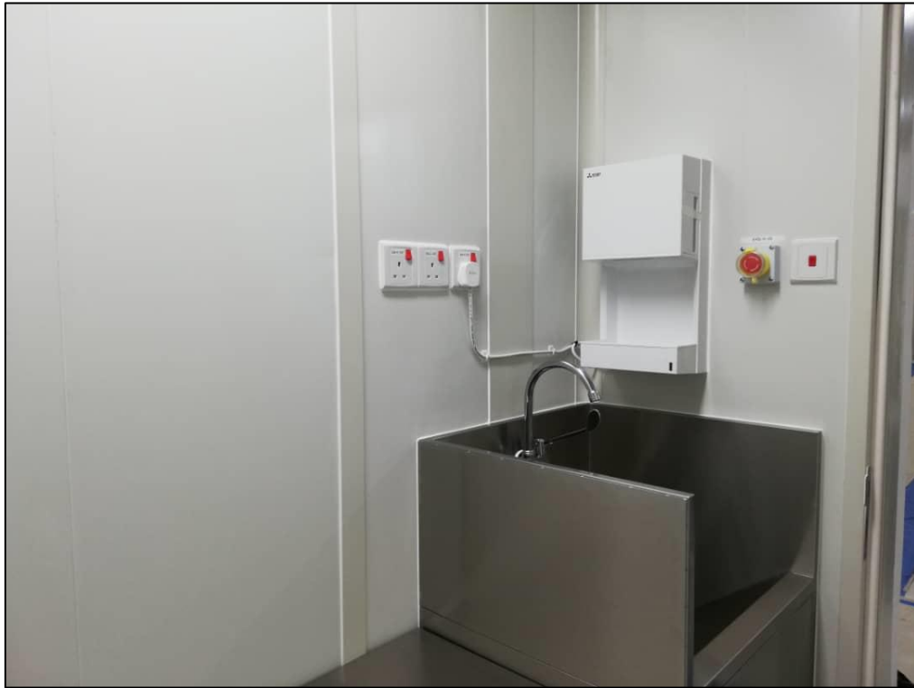
Image 19: QC Room Internal Site Condition (View 3)
