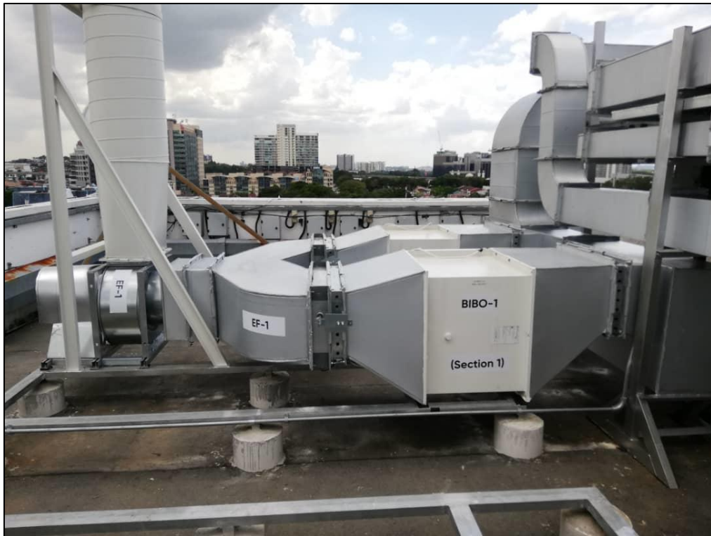
Image 30: Rooftop Site Condition (View 1)
