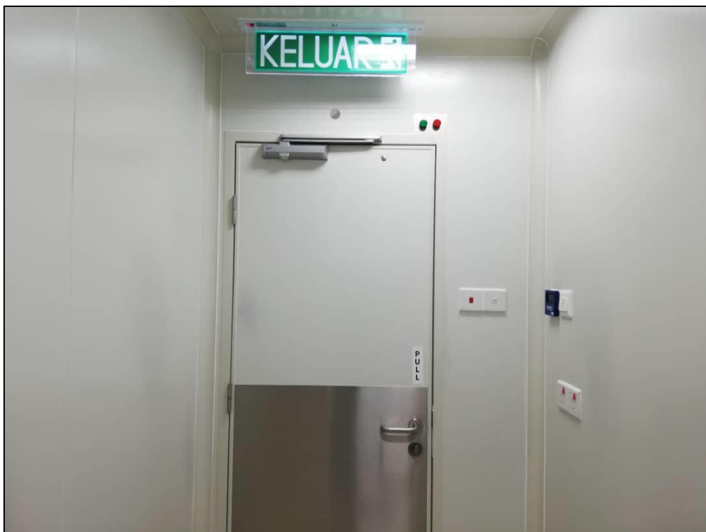
Image 28: Transfer Room Internal Site Condition
