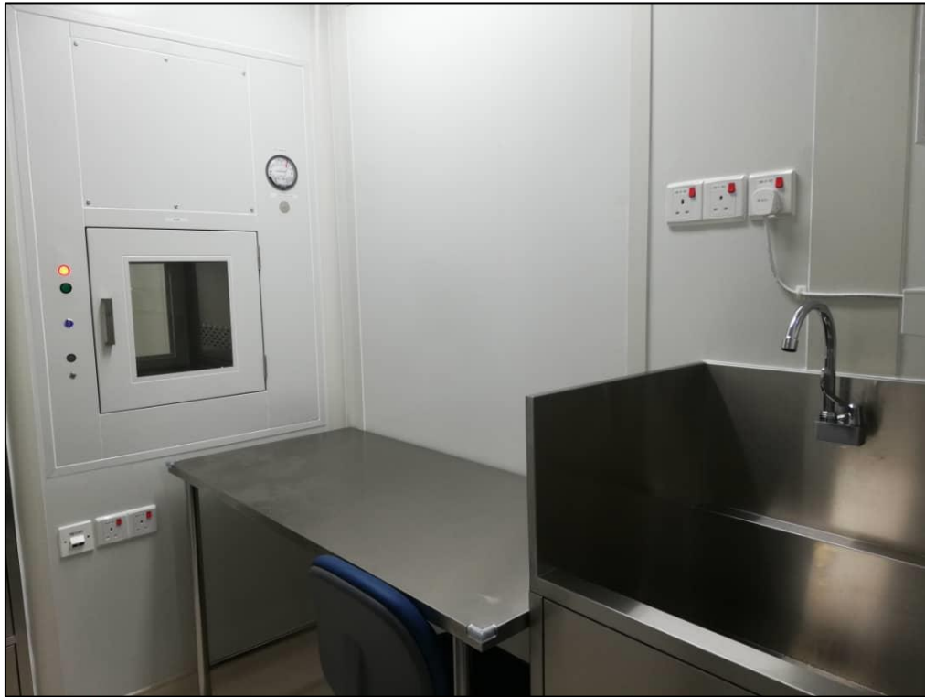
Image 17: QC Room Internal Site Condition (View 1)
