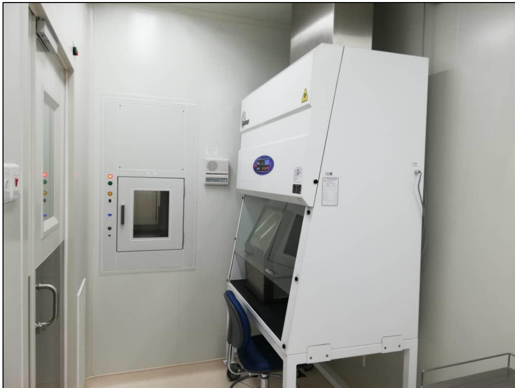
Image 26: Radioiodine Room Internal Site Condition (View 2)
