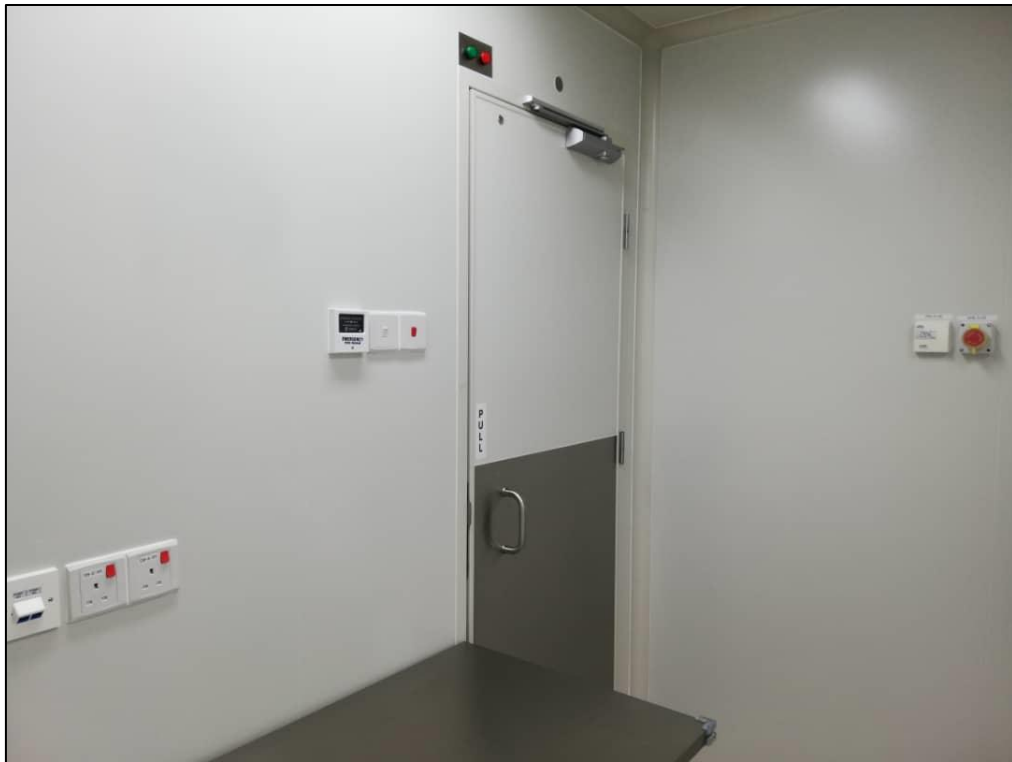
Image 14: Component Preparation Room Internal Site Condition (View 1)
