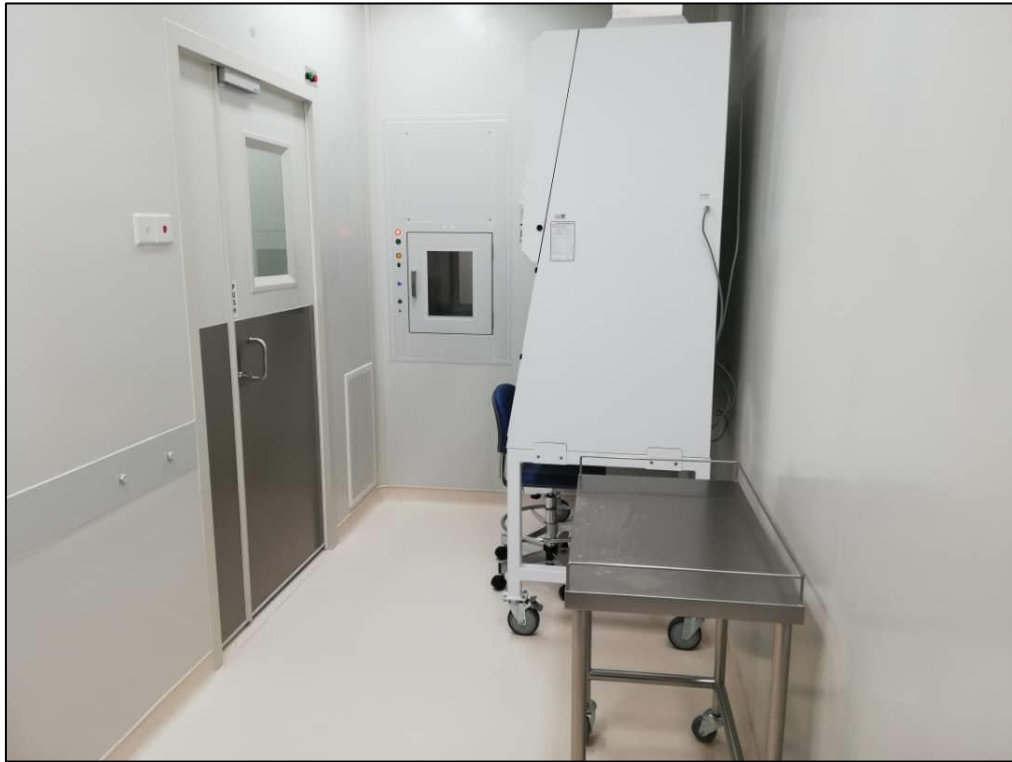
Image 25: Radioiodine Room Internal Site Condition (View 1)
