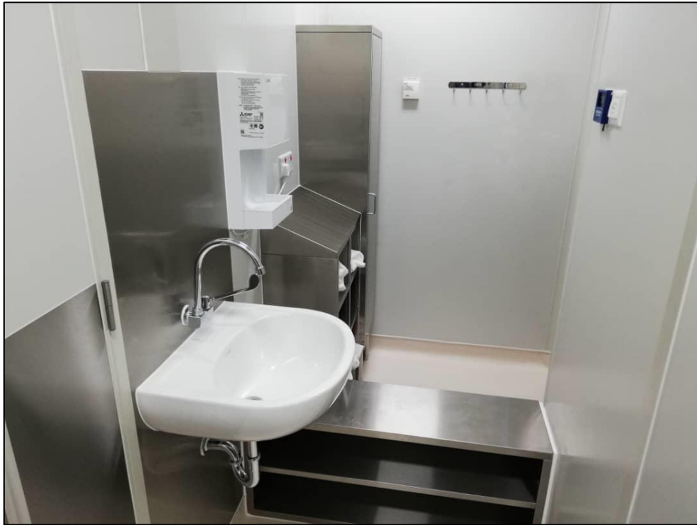
Image 23: Change Room 2 Internal Site Condition (View 1)
