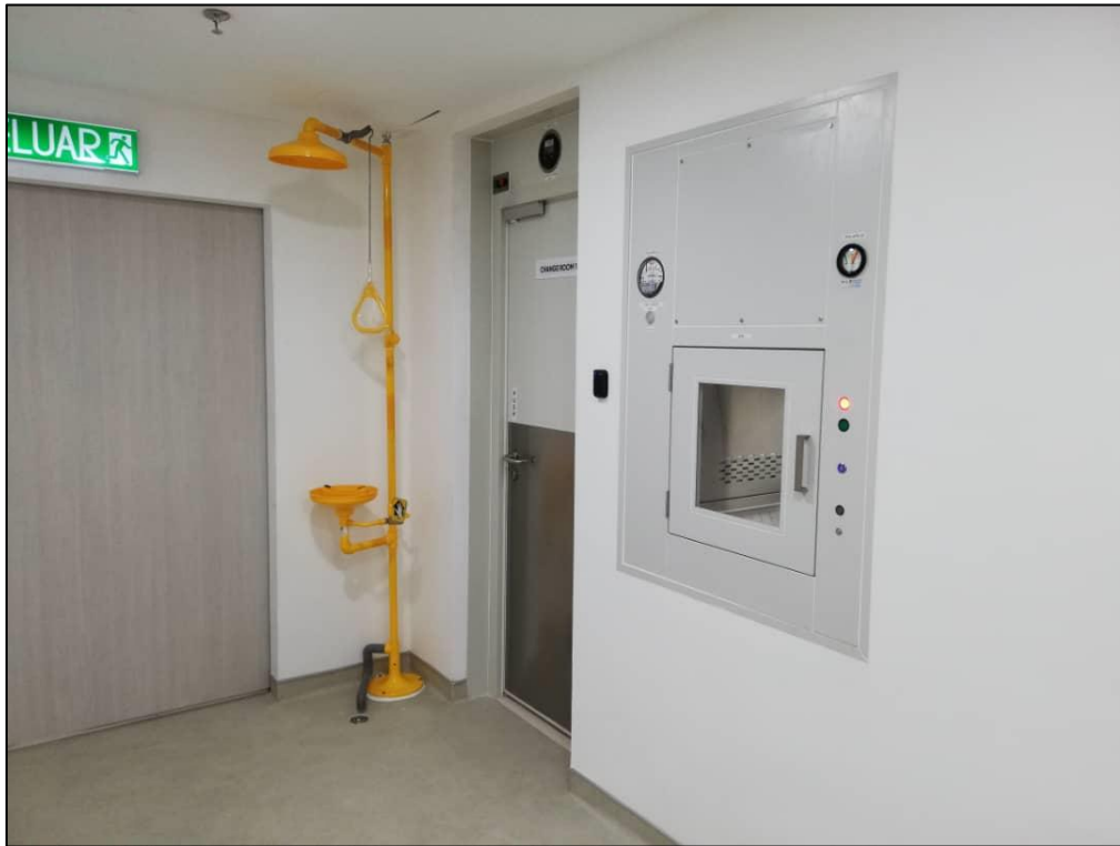
Image 21: Nurse Station Site Condition (View 2)
