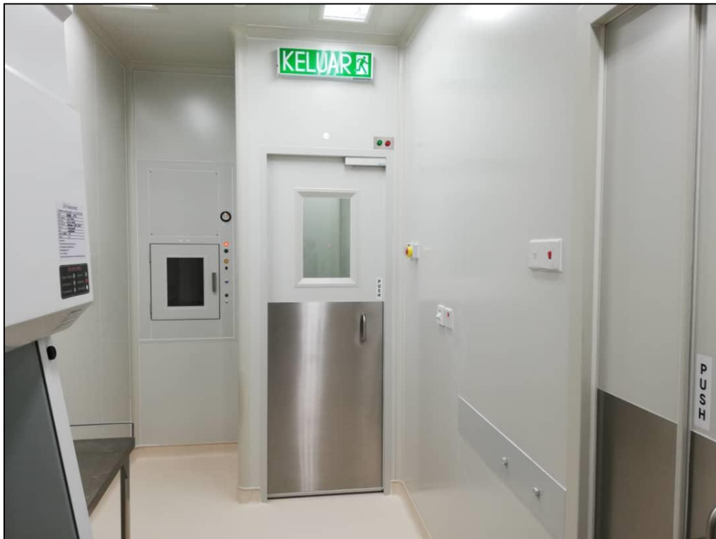
Image 27: Radioiodine Room Internal Site Condition (View 3)
