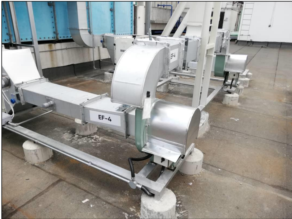
Image 31: Rooftop Site Condition (View 2)
