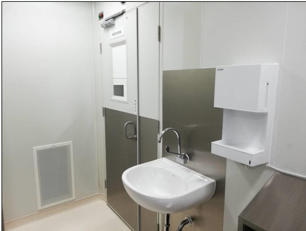
Image 24: Change Room 2 Internal Site Condition (View 2)
