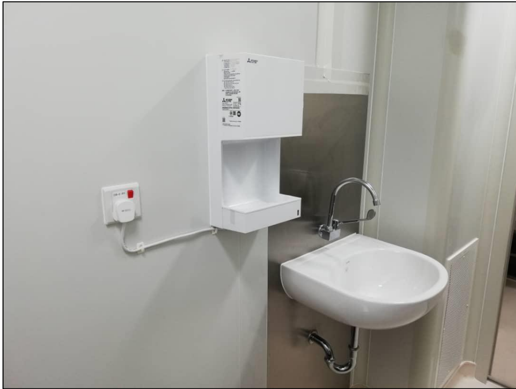
Image 13: Change Room 1 Internal Site Condition (View 3)
