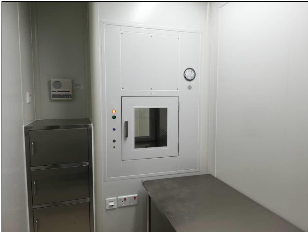
Image 18: QC Room Internal Site Condition (View 2)
