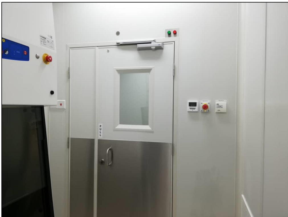
Image 2 – SPECT/CT Hotlab Internal Site Condition (View 2)
