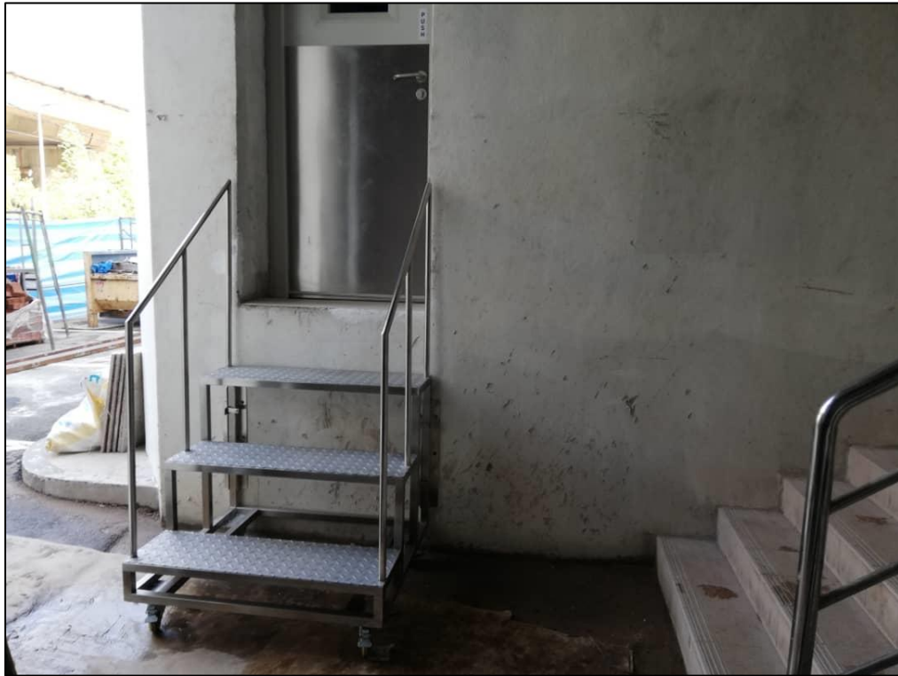
Image 29: Decay Room External Site Condition
