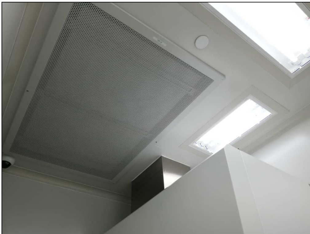
Image 8: PET/CT Hotlab Internal Site Condition (View 3)
