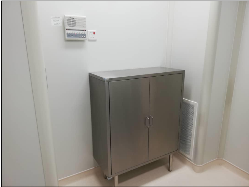
Image 15: Component Preparation Room Internal Site Condition (View 2)
