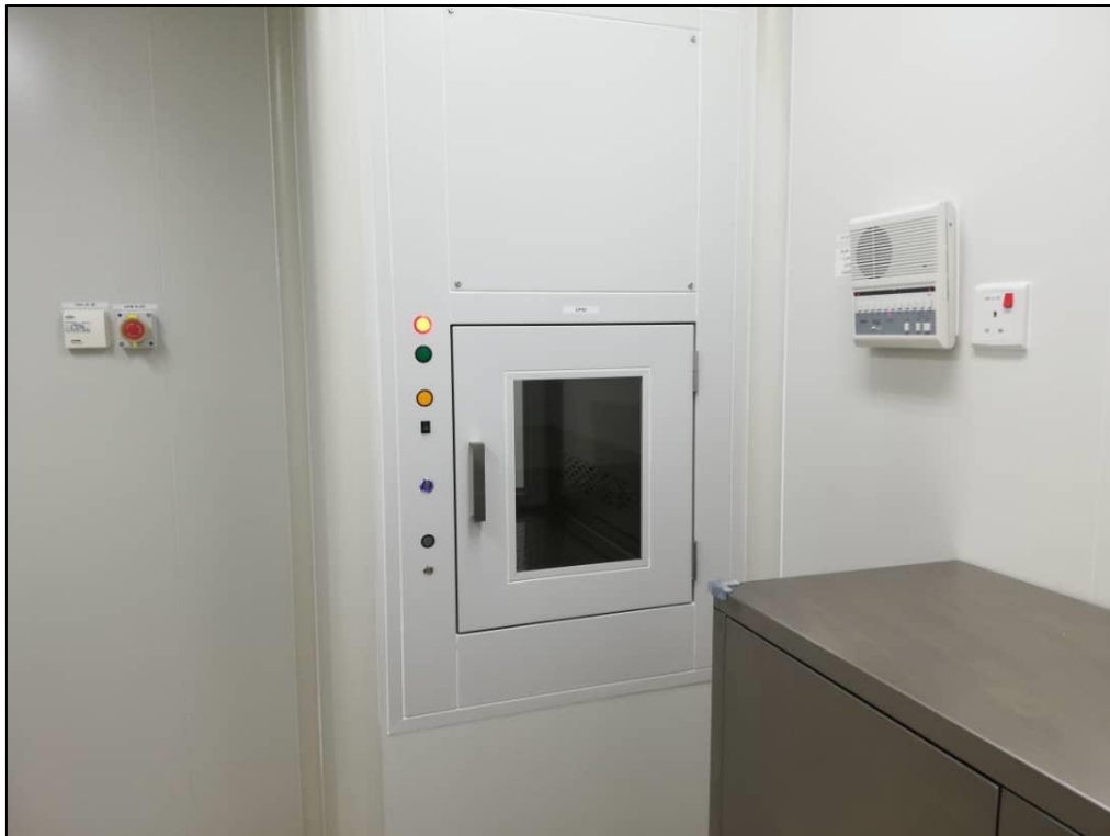
Image 16: Component Preparation Room Internal Site Condition (View 3)
